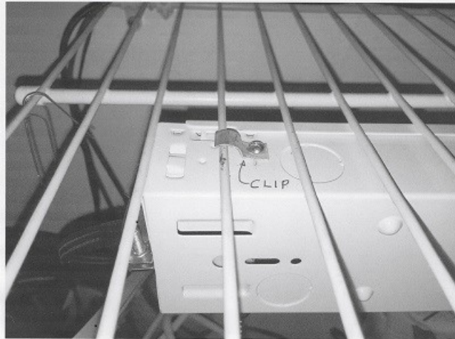
CLIP ATTACHES LIGHT FIXTURE TO WIRE SHELF
